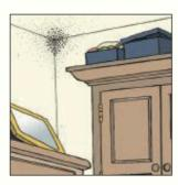
Condensation is caused by water vapour or moisture from inside the dwelling coming into contact with a colder surface, such as a window or wall. The resultant water drops (condensation) may then soak into the wallpaper or paintwork or even plasterwork. In time, the affected damp areas then attract black mould that grows on its surface.
